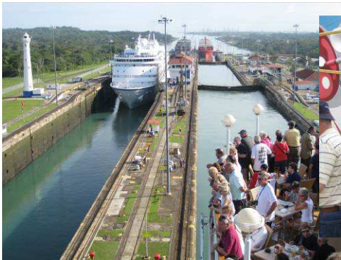
Panama Canal, an engineering marvel (parts are orig. date back 1914)
