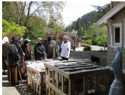
Restoration of Our Lady's statue and Fountain in work.
