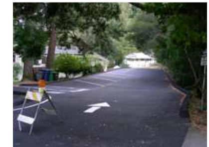
New asphalt at St. Cecilia's
